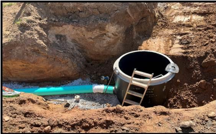
Tomco Installing Sanitary Sewer Line Manhole
