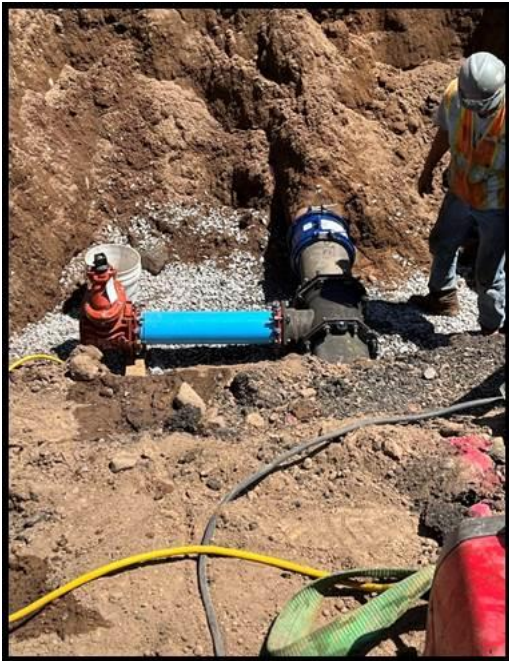
Tomco Connecting Water Pipe to Water Source
