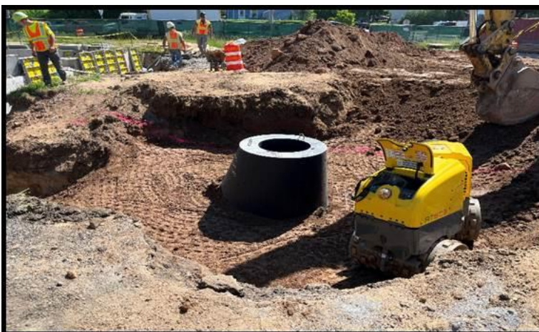
Tomco Crew Installing Water Line Vault
