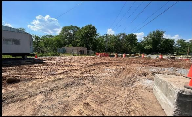
Tomco Completed Backfilling Soils
