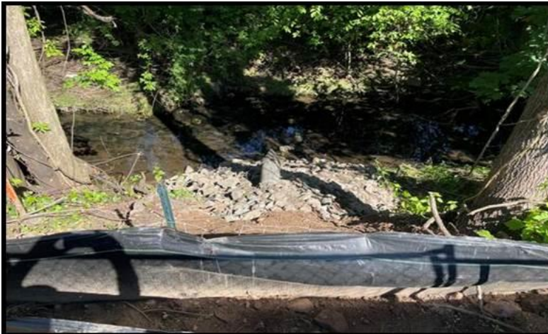
Tomco Placed Stones to Prevent Soil Runoff
