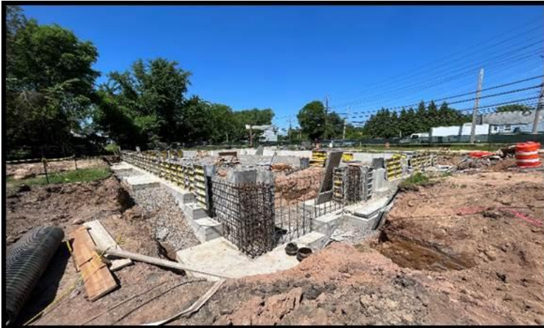
JR Prisco Completing Form Building East Side Foundation Wall
