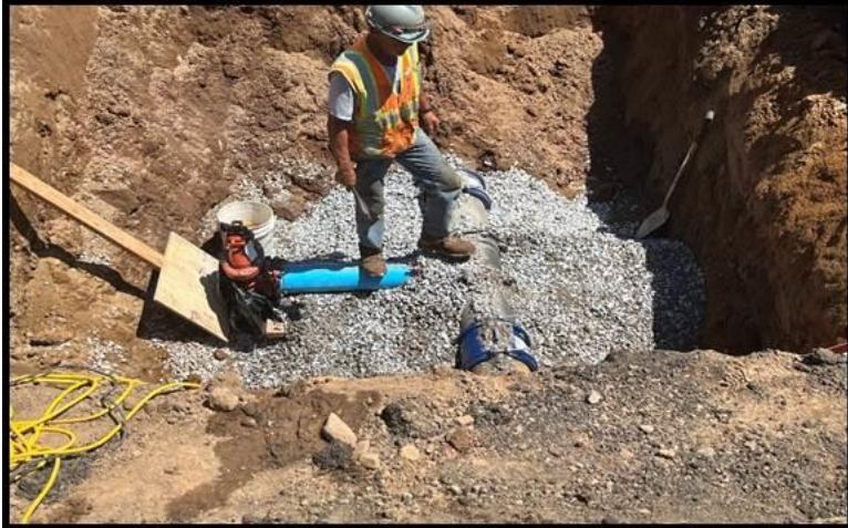
Tomco Backfilling Gravel Around Waterline
