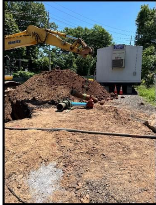
Tomco Installing Water Pipe Connection
