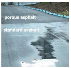
Porous asphalt vs. Standard asphalt.
