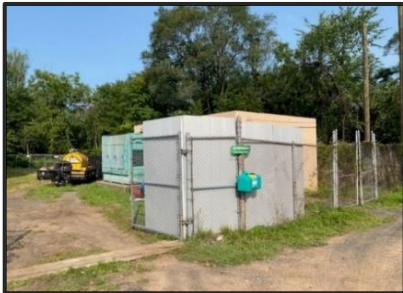
Foam boards to reduce noise from generator.
