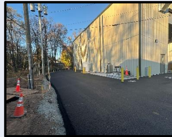
Paved Driveway Westside Building
