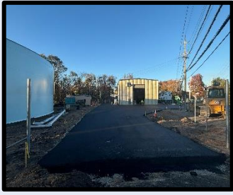
Paved Driveway Looking North
