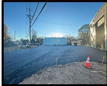
Paved Driveway Looking West
