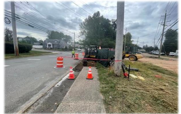
Curb Removal for Installing of New Curb Cut Out
