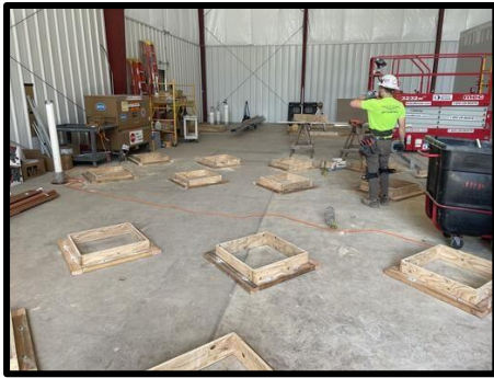
Indoor Concrete Pad Framing
