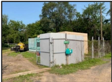
Foam boards to reduce noise from generator
