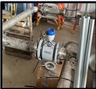
Flow Meter Install
