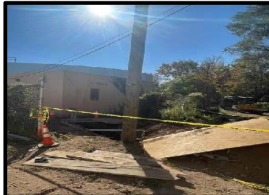
New Electrical Pole Installed near FL House
