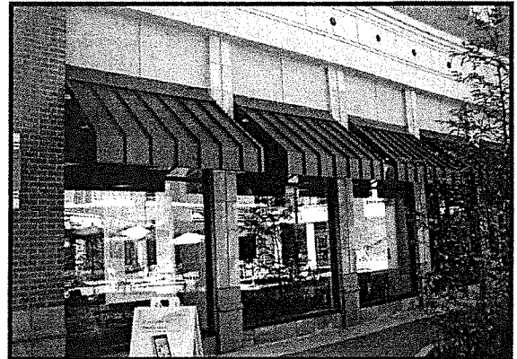
Awnings provide screening from the sun and provide architectural dimension.
