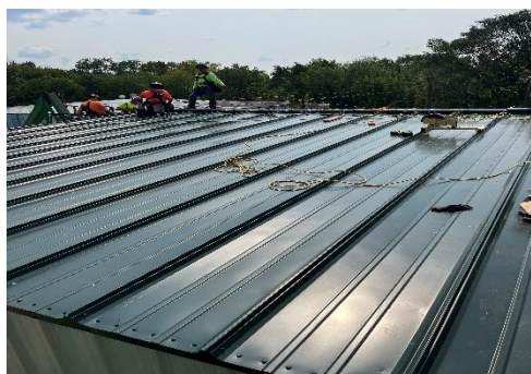
Building Roof Installation
