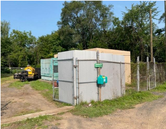
The foam boards around the fence near the generator that will help reduce noise during operations.
