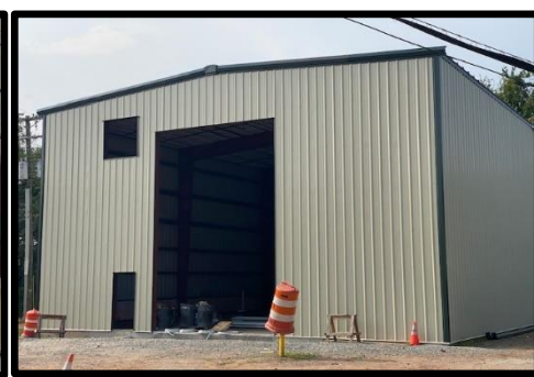
Building Roof Complete South Side View
