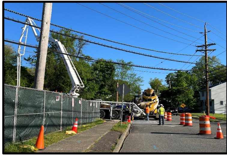
Concrete Truck Loading Pumper
