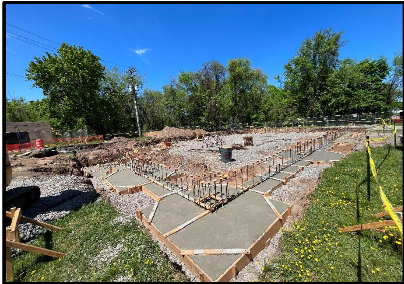
Finished Concrete Footings
