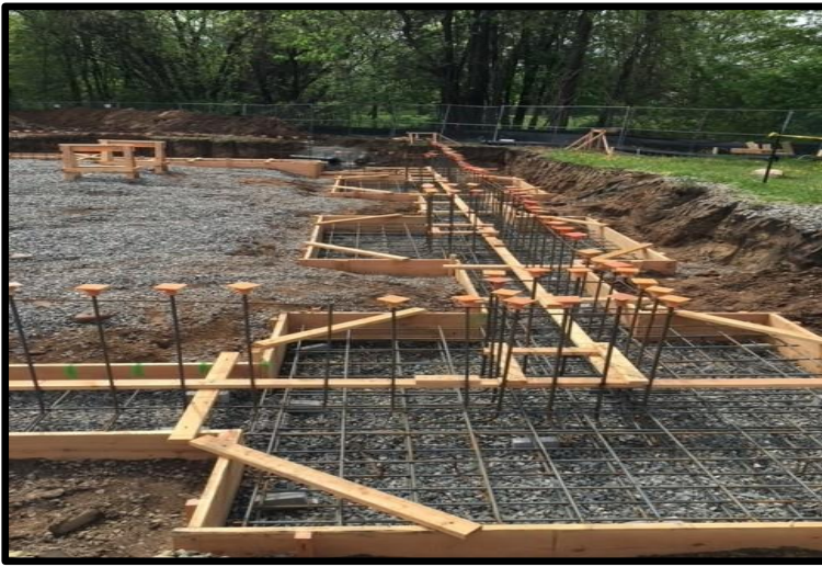
Concrete Rebar Footings
