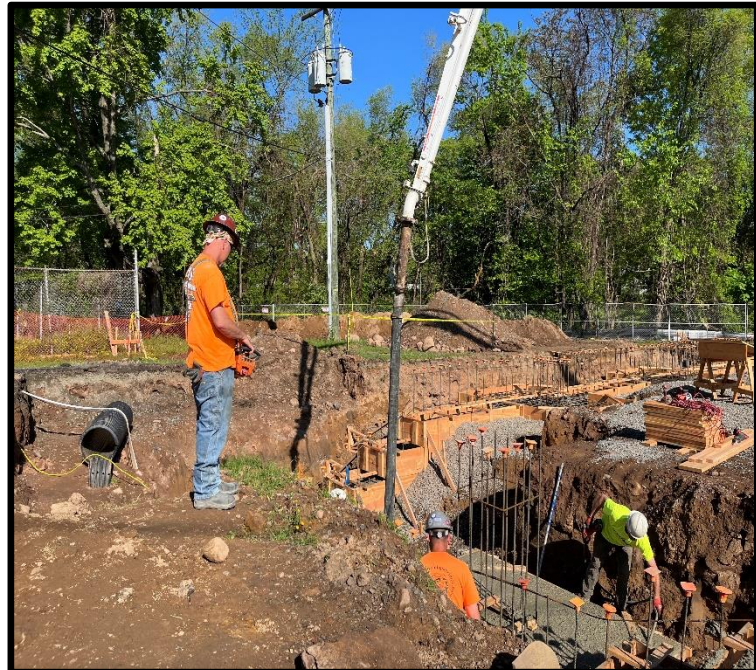
Pouring/Pumping Concrete into Foundation Footings
