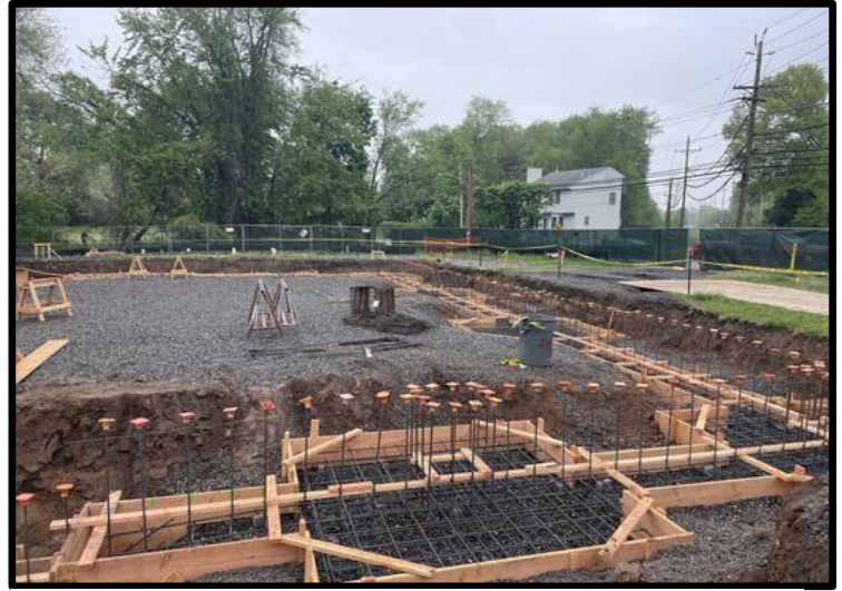
Foundation Rebar Footings
