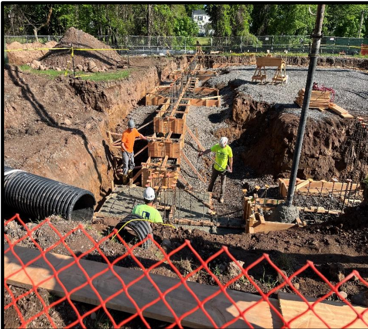
Pouring/Pumping Concrete into Footings
