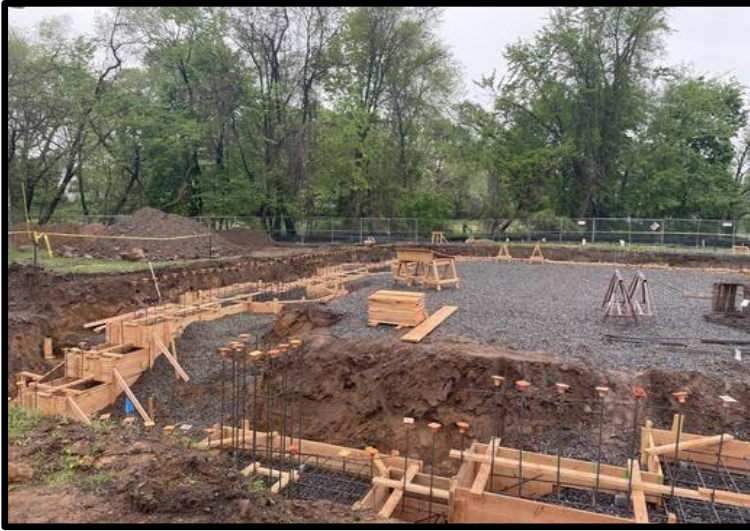
Finished Foundation Rebar Footings
