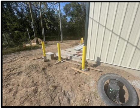
Bollards Installation
