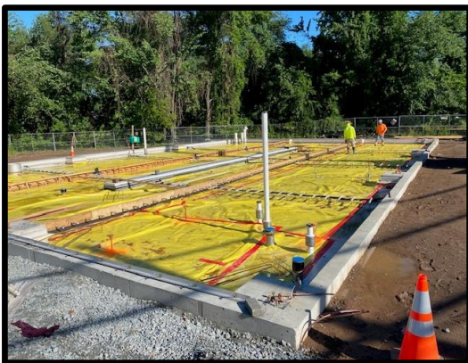
JR Prisco inspecting the wood forms before pouring concrete
