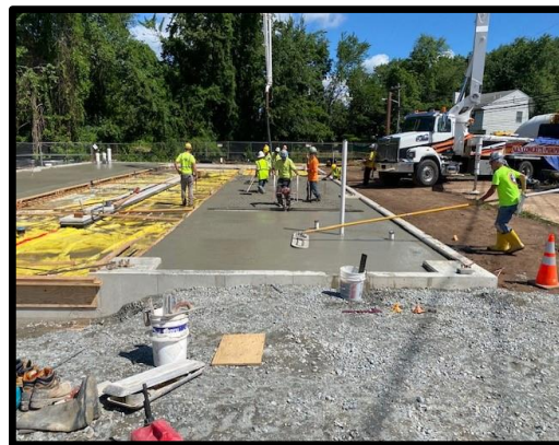
JR Prisco pouring concrete on the eastside slab/floor
