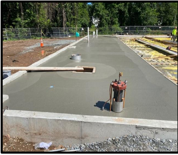
Finished Concrete Slab/Floor West Side
