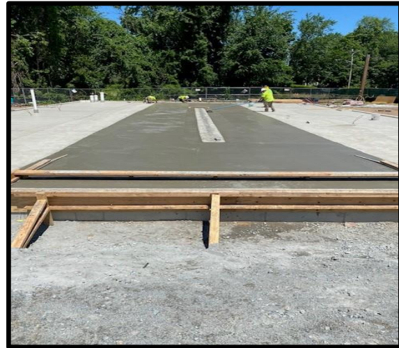
Finished Center Slab/Floor Concrete
