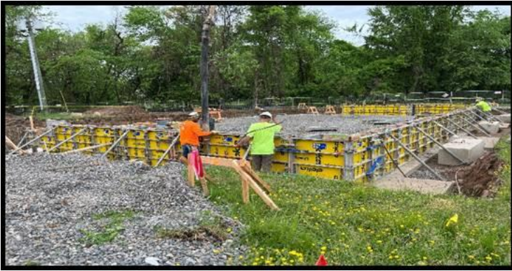
JR Prisco Crew Pouring Concrete Foundation Wall East
