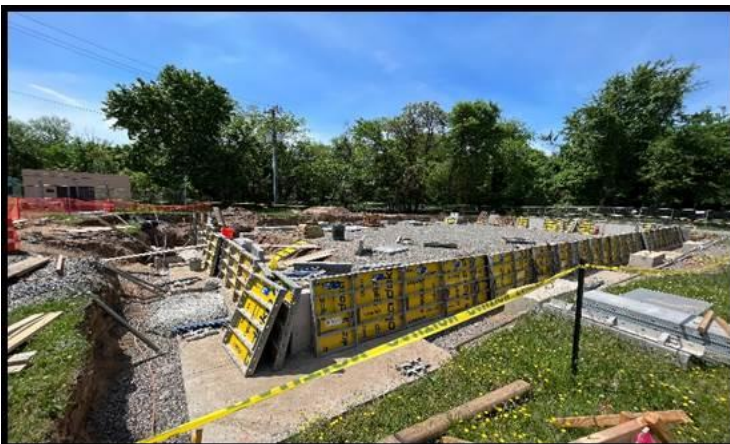
JR Prisco Removing Building East Side Foundation Wall
