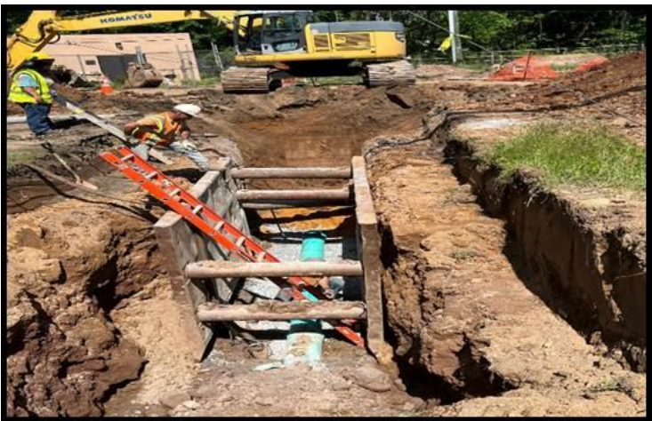
Tomco Installing the Sewer Water Pipe
