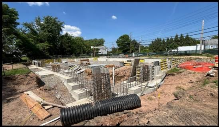
JR Prsico Building Foundation Wall West Side of Treatment Plant
