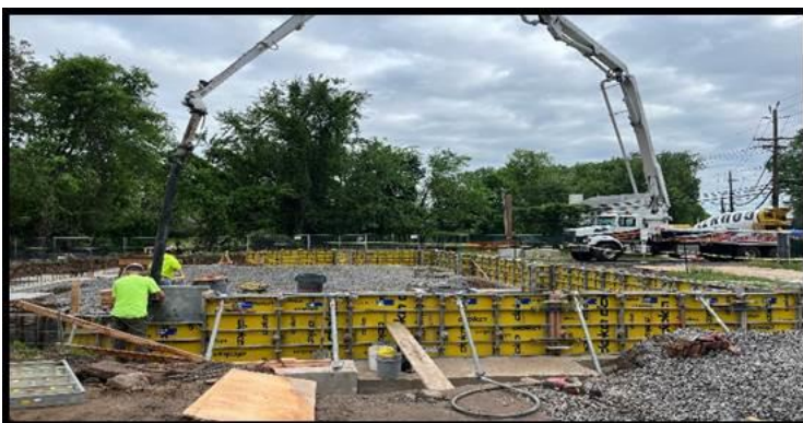
Foundation Wall East Pumping Concrete
