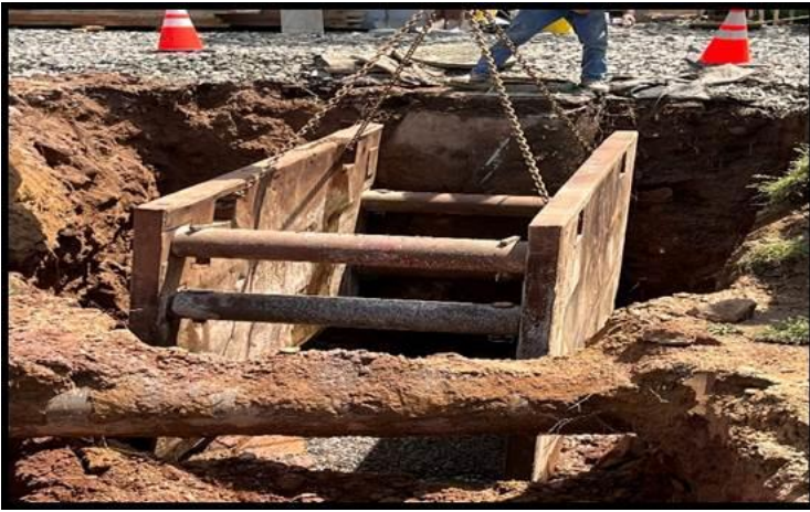
Tomco Setting Trench Box for Sewer Pipe Install
