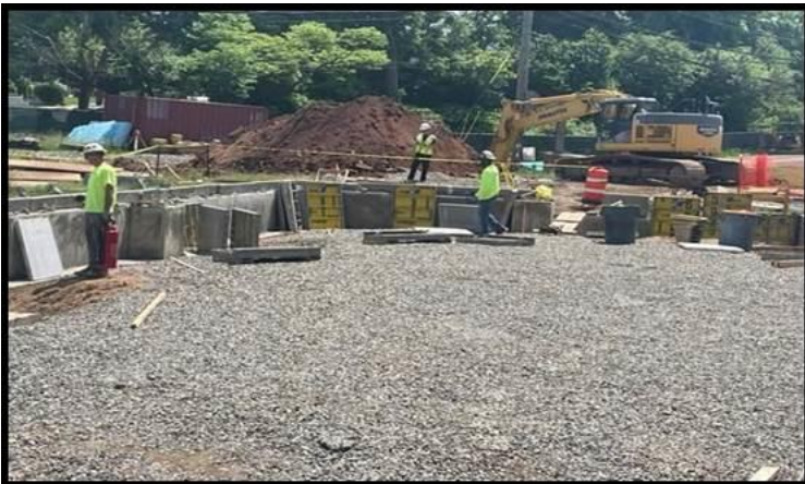
JR Prisco Removing Forms/Panels East Side Treatment Building
