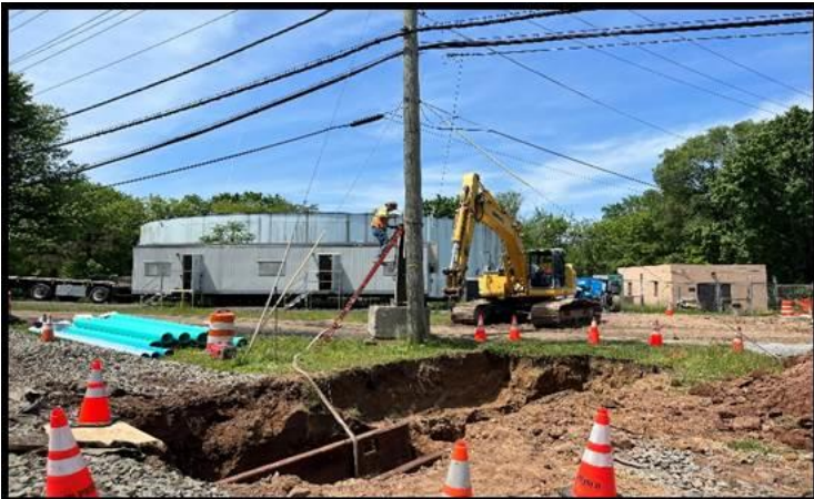
Tomco Stabilizing Electric Pole During Sewer Pipe Excavation
