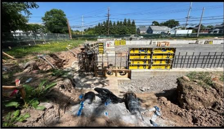
JR Prsico Building West Side Foundation Wall Near Water Pipe Entrance
