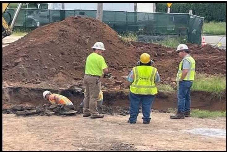
PSEG and Transco Observing the Sewer Pipe Installation
