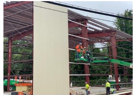
Building Metal Siding Installation Begins
