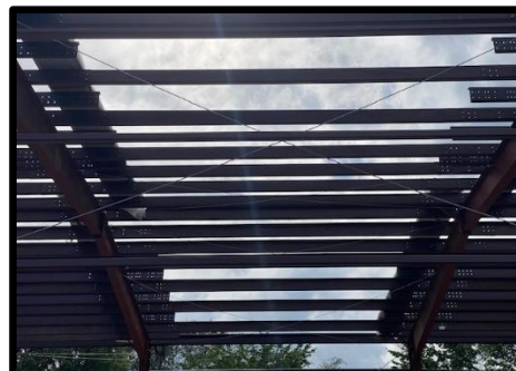
Finished PEMB Roof Joists
