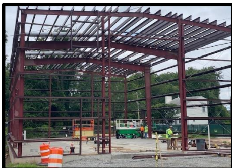
Finished PEMB Structural Frame
