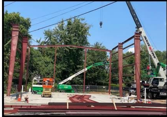
Day 2 Metal Building Construction
