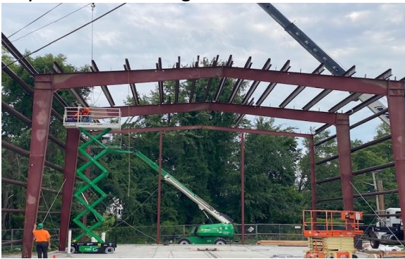
Day 3 Metal Building Construction
