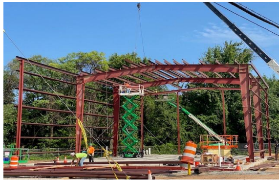
Day 3 Metal Building Construction
