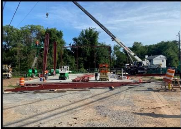
Day 2 Metal Building Construction
