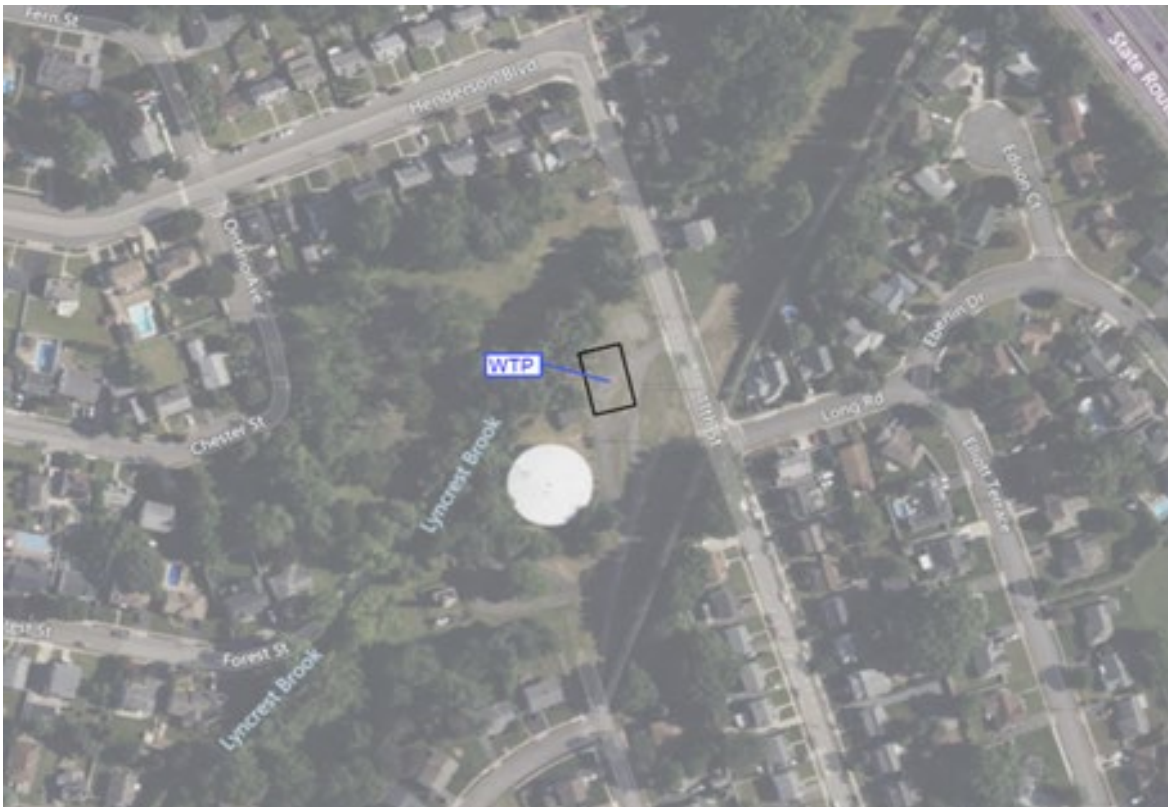
Location of the new groundwater treatment facility along 11 th Street in Fair Lawn, New Jersey. Shown here as a blue rectangle.
